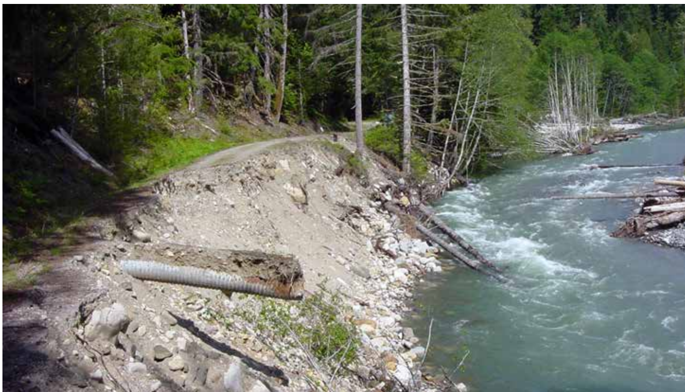
A washout on the Suiattle River Road—milepost 20.8—about a tenth of a mile west of the Downey Creek Bridge
