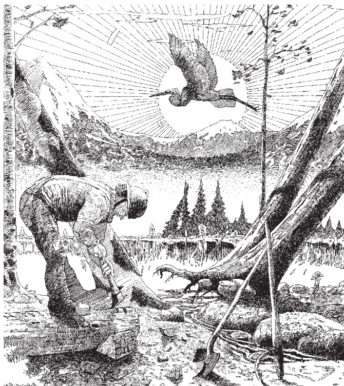
Cutting a flat surface onto a log for bridge construction. Illustration by SCA crew leader Peter Lucchetti.
