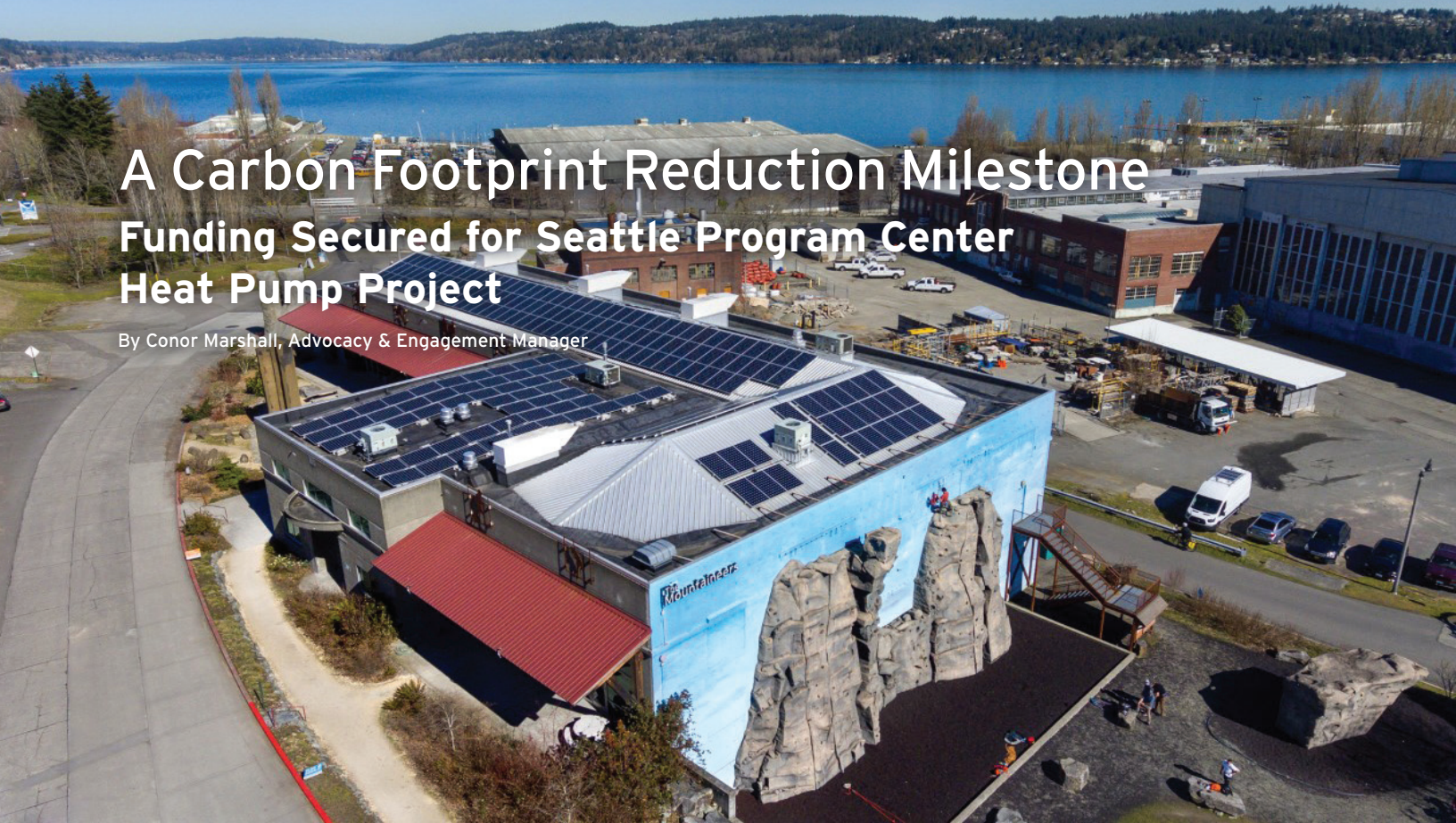
Solar panels on the Seattle Program Center (SPC) roof. Transitioning to energy-efficient heat pumps represents a major step toward achieving net zero carbon emissions for the SPC. All photos courtesy of the Carbon Footprint Reduction Committee.
